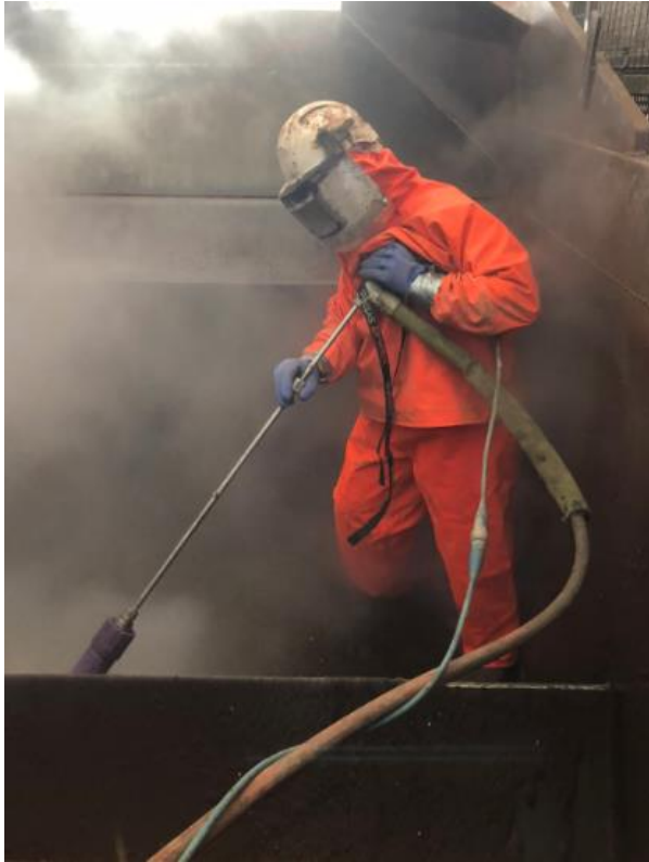
Figure 2. Cleaning with a high-pressure water jet. hydroblast.co.uk (n.d.)
