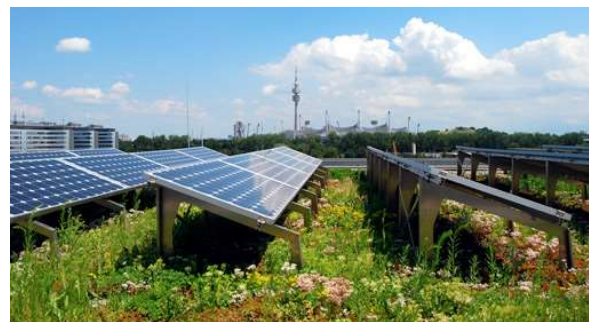
Figure 1 A reference image of a green roof combined with PV panels. (Greenscape, 2017)
