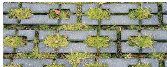
Figure 3 Reference image of porous paving materials as is implemented in EVA-Lanxmeer. (Author, 2017)
