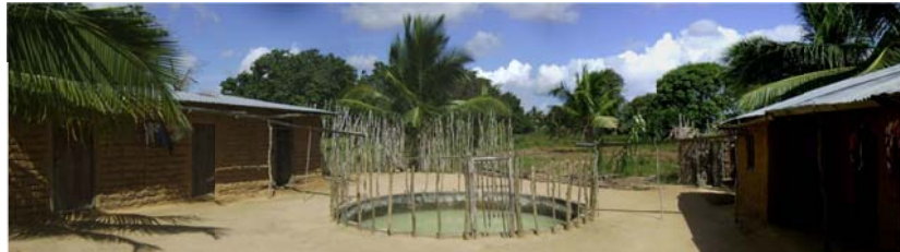
Figure 4.4 Reservoir in Malamba, where water from two roofs and from the surface are collected for filling the tank. A fence of wood is constructed to prevent falling in. A small door, in the front, give access to the water
