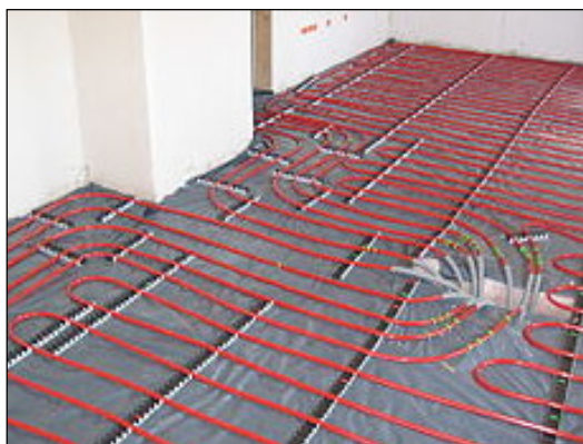
Figure 10 - Hydronic radiant floor
