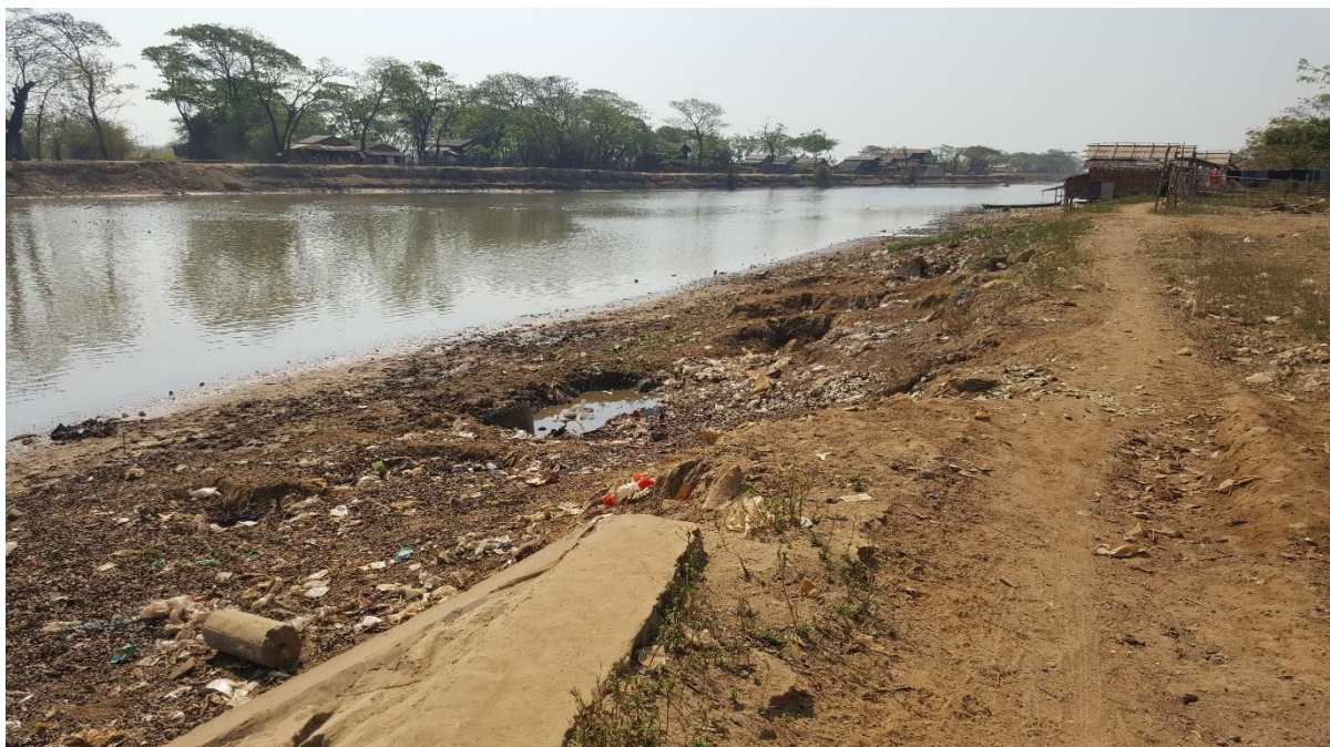
FIGURE 15: EROSION ON THE DRAINAGE CANAL DIKE NEAR THE MINYWA SLUICE GATE
