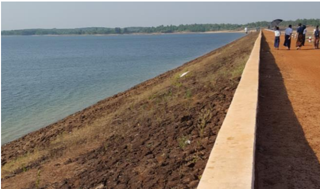
FIGURE 7: THE MAZIN DAM IS COATAD WITH LAVA STONE
