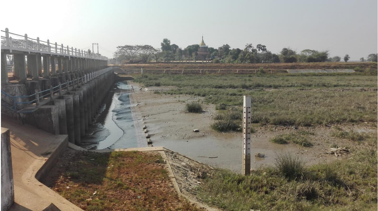
FIGURE 5: THE TAWA SLUICE GATE, SEDIMENTATION DIRECTED FROM THE OCEAN IS CLEARLY VISIBLE A METER FROM THE GATES
