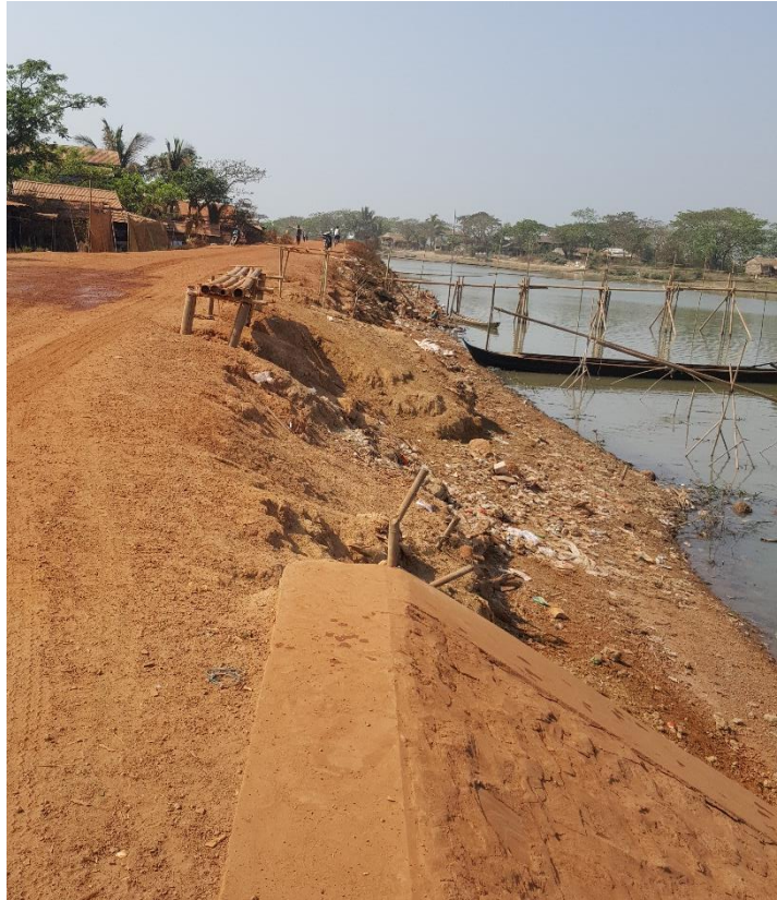
FIGURE 14: EROSION ON THE BAGO-SITTAUNG CANAL DIKE NEAR THE MINYWA SLUICE GATE
