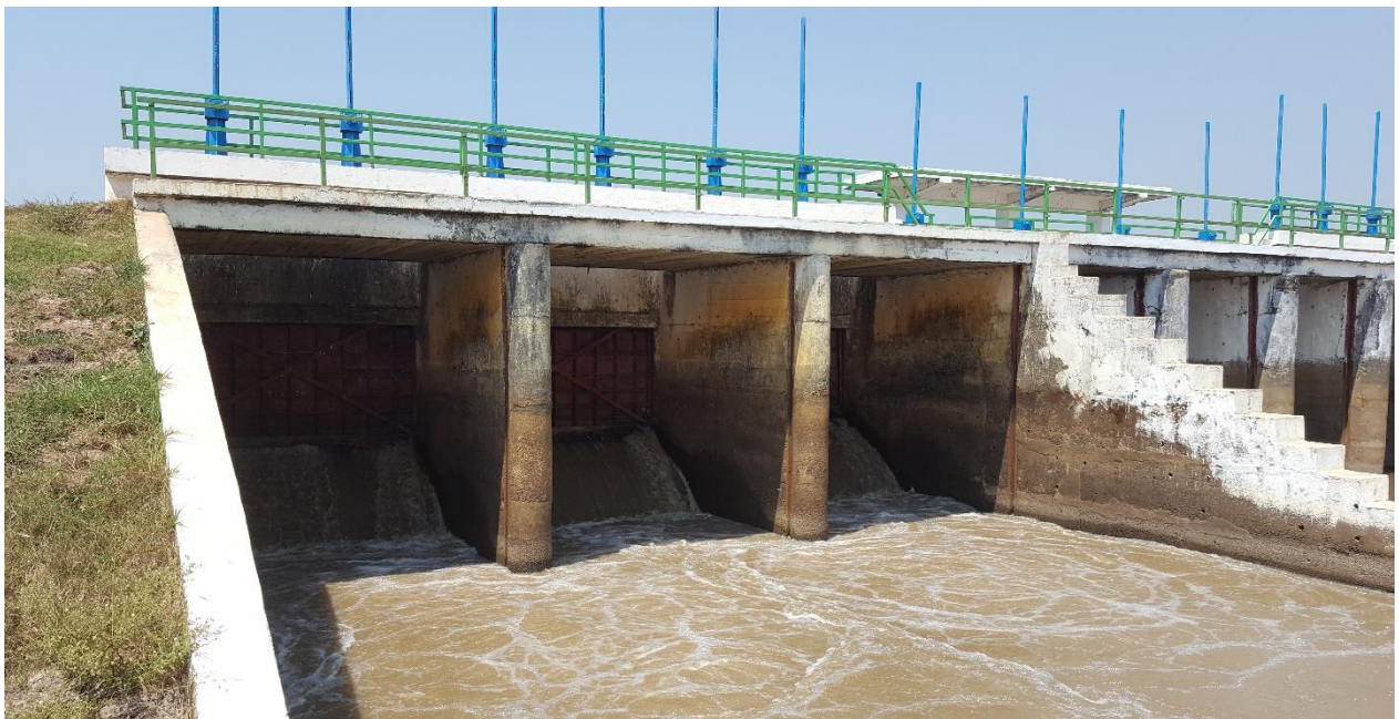
FIGURE 18: ONE OF THE TWO OUTLETS OF THE MOE YIN GYI LANK RESERVOIR, THE MOEYINGI SLUICE GATE
