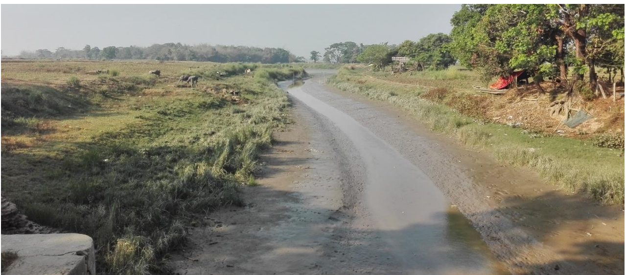
FIGURE 5: SILT CLEARLY VISIBLE ON THE BAGO-RIVER SIDE OF THE SLUICE
