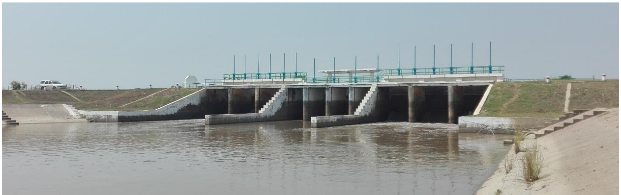
FIGURE 17: ONE OF THE TWO OUTLETS OF THE MOE YIN GYI LANK RESERVOIR, THE MOEYINGI SLUICE GATE
