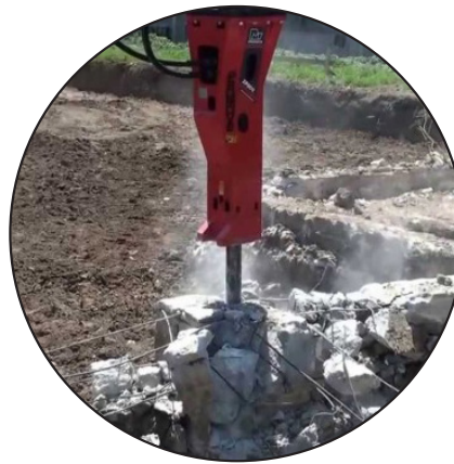
Removing old foundations
