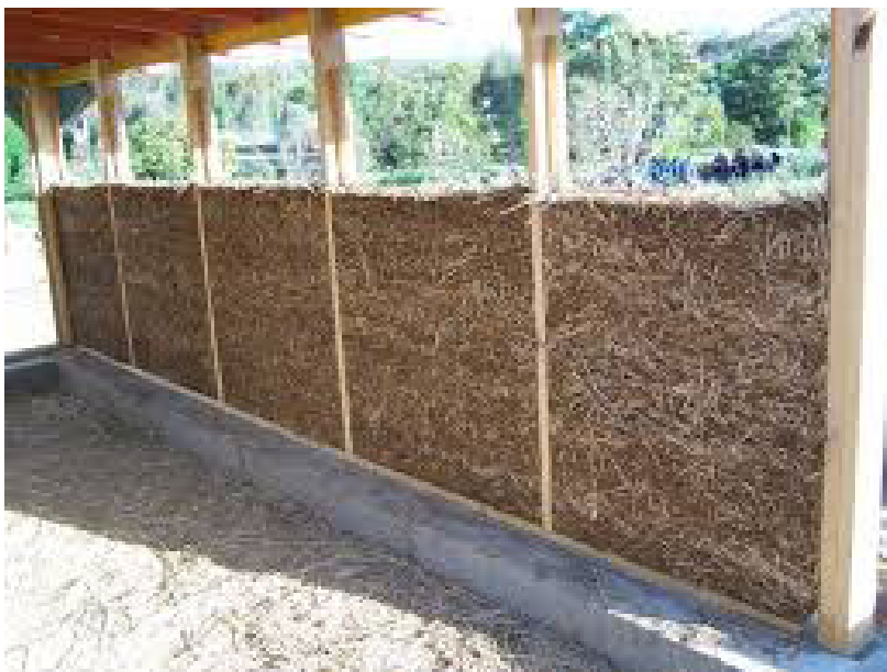
figure 10: Straw light clay building method example, source: (Handersen, 2014)
