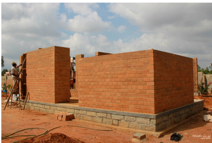
figure 11: CSEB building method example, source: (Made in Earth, 2015)
