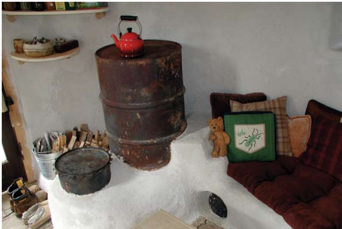
Above: Chris Reinhart's Rocket Stove. Note that the barrel is exposed quite a bit to maximize radiant heat. Below: Kirk Mobert's Rocket Stove with cooking surface on top. There are two cold air intakes below the metal door. The cob bench box keeps firewood dry.
