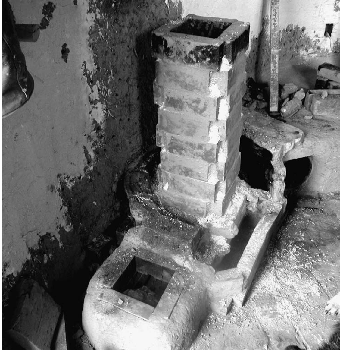
A good example of a brick tower under construction in Chris and Jenn Reinhart's house. A fortress of brick is mortared in to support the barrel. Photos, this page: Chris Reinhart.
