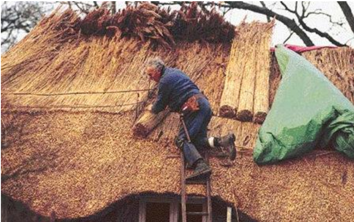
Figure 11: Roof thatching with common reed ( P. australis ) (Fewins, 2000)
