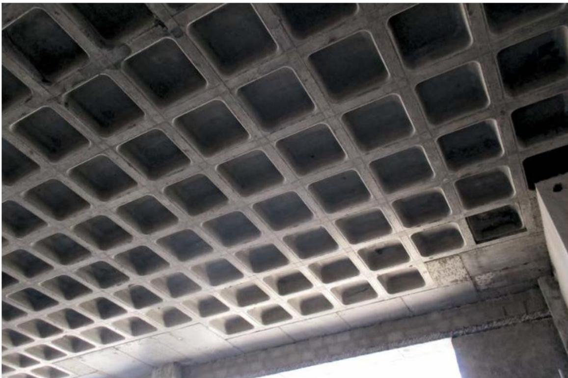
Figure 2 - example of reticular slab
